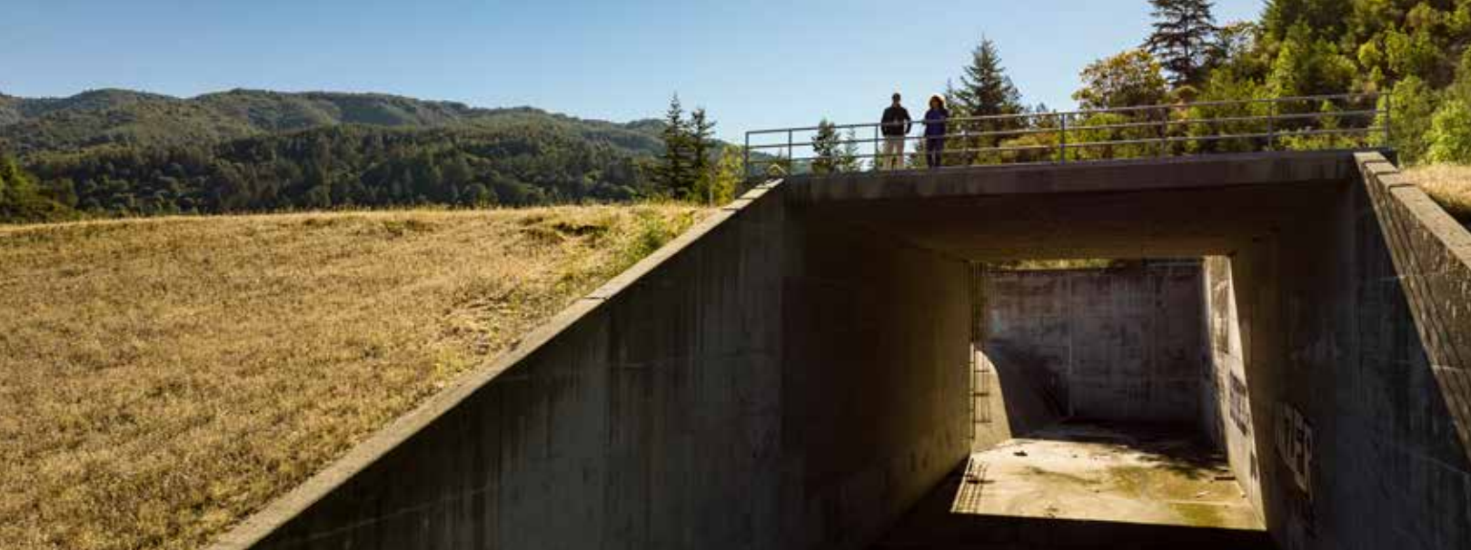
San Jose Water Staff at Austrian Dam.
